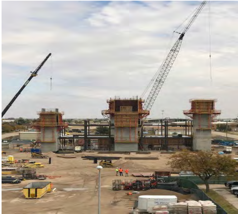
Construction of the new Judicial Complex
